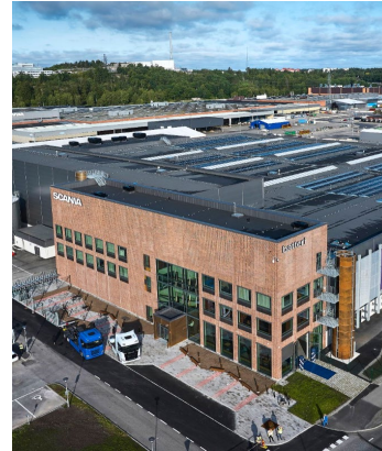
Scania's battery assembly starts operations
