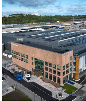
Scania's battery assembly starts operations
