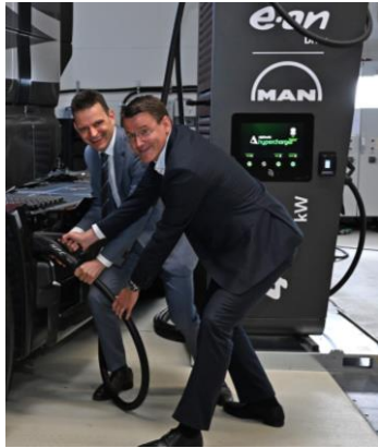
MAN and E.ON build public charging network in Europe
